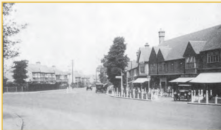
‘Shirley Park Parade shortly after construction in 1928’
