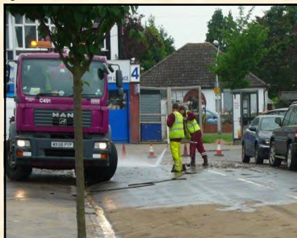
High pressure hose used to wash away the mud slurry
