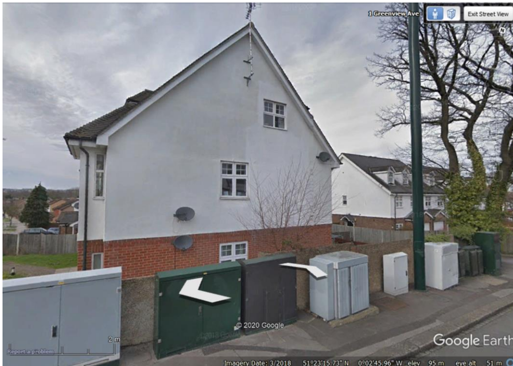
Google Earth image of Mast Position and street cabinets at March 2018
